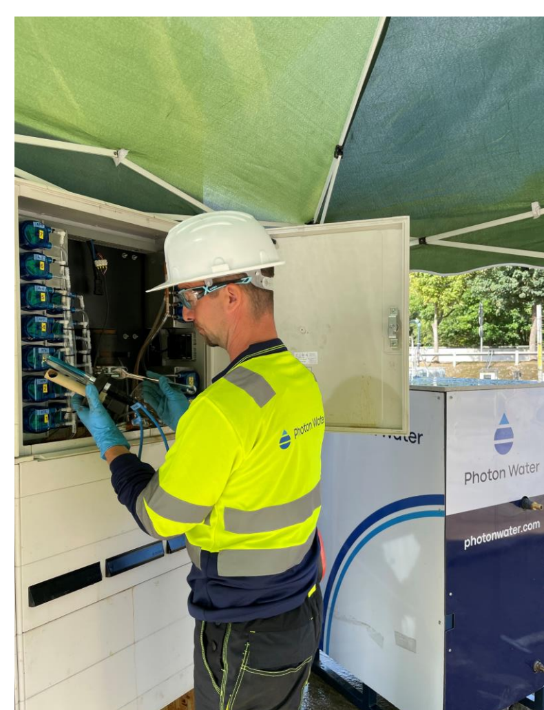
Figure 5: Groundwater Sampling Unit for sampling all piezometers
