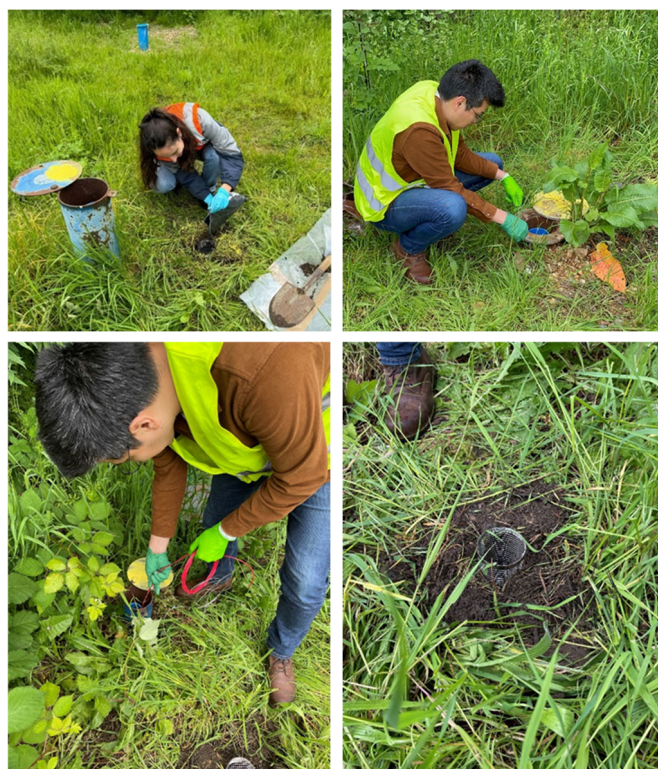
Figure 8. Installation of the electrodes at the site in the UK.
